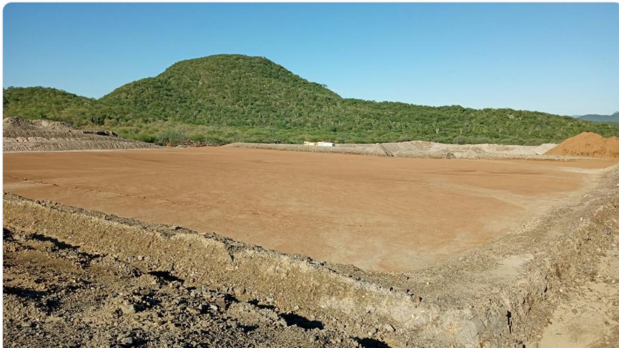
Photo: the permitted 50,000-tonne heap-leach pilot plant at Gran Pilar (Sonora, Mexico) – the prepared heap-leach pad, the Sierra in the background. Source: Tocvan Ventures Corp.
